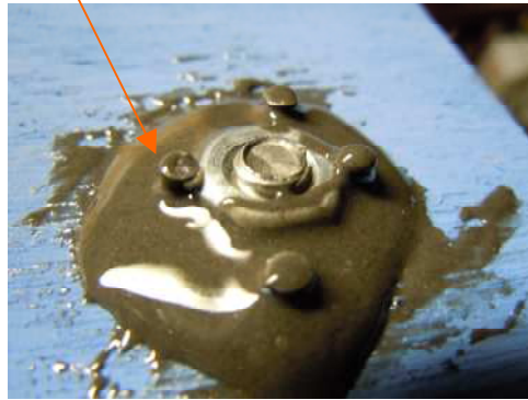
Epoxied nuts Small nails to help hold epoxy to board and nut
